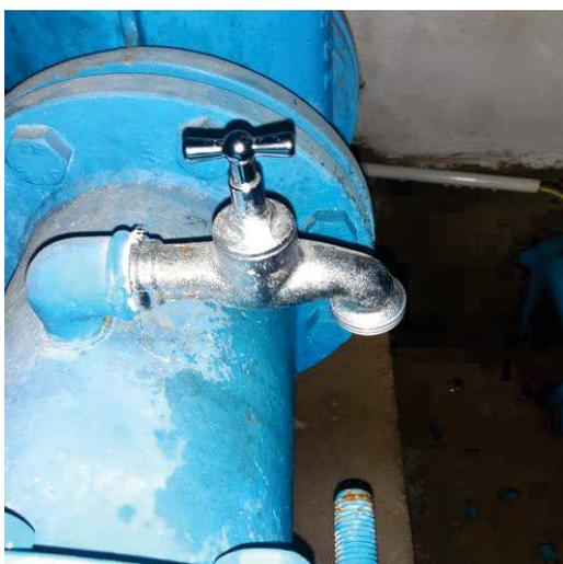
Abb 7: HB Kammern – PN-Hahn (innere Kammer)
